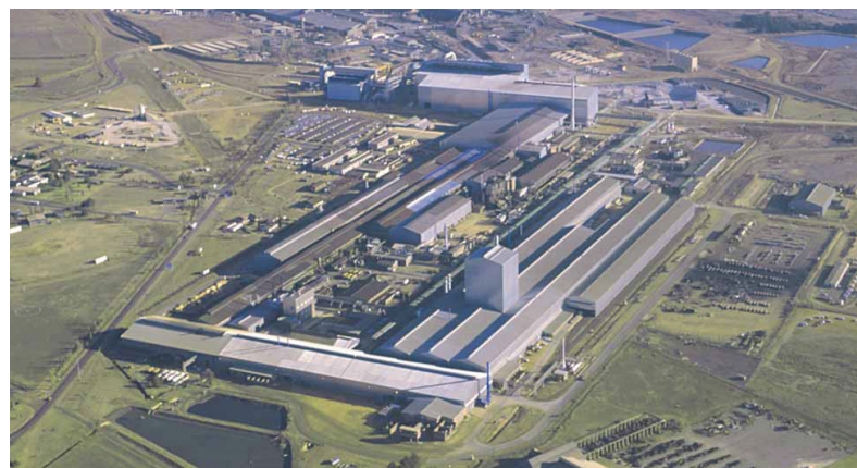
Columbus Stainless steel plant in South Africa
