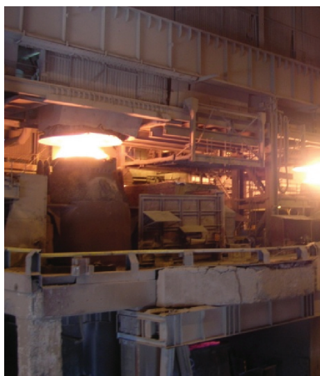
Fig 1 Columbus twin 120t AOD converters operating with steam as a process gas
