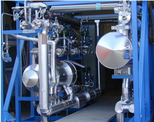
Figure 1. Heat exchangers and insulated pipes in steam/AOD-gas mixing station.
